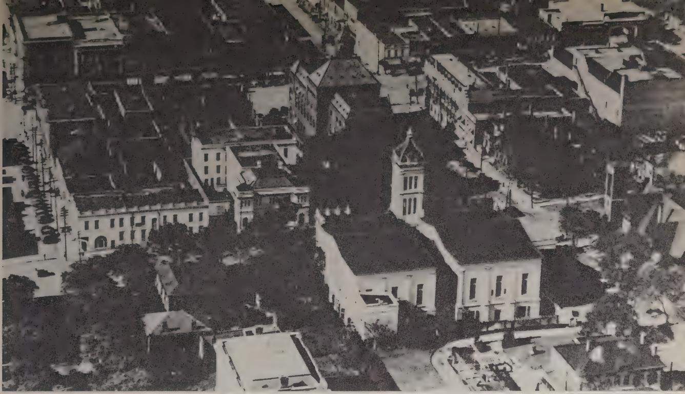
Aerial view showing the rear of the Court House from Adams Street looking North and East in 1930.
